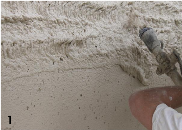
Applying the surface
