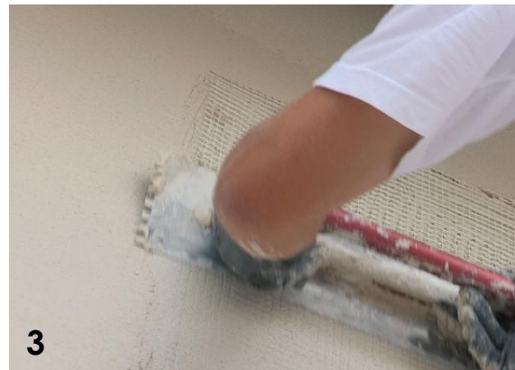
Embedding the reinforcing mesh
